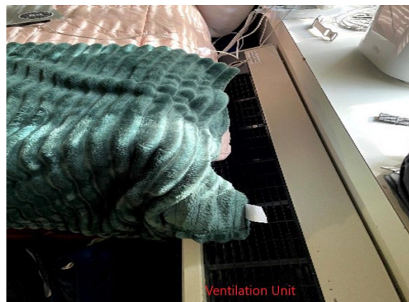
Example of bed and bedding too close to the ventilation unit. Allow as much open space as possible around the unit.
