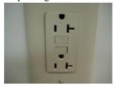
Power to the device should be restored when the reset button is pushed. If the GFCI is found to be defective, discontinue use of the outlet and label it "Defective-Do Not Use" and contact your building
