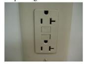
should shut off. Power to the device should be restored when the reset button on the outlet is pushed. If the GFCI is found to be defective, discontinue use of the outlet and label it
