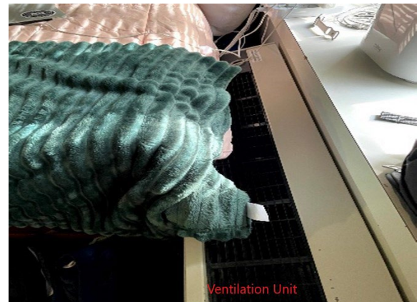
Example of bed and bedding too close to the ventilation unit. Allow as much open space as possible around the unit.
