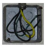
Electrical components including switches, outlets, junction boxes, wire raceways, circuit breaker panels, etc. must be guarded to prevent accidental contact with live electricity. If you observe exposed wiring,
