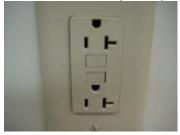
A ground-fault circuit interrupter (GFCI) is a device that is designed to quickly detect a ground fault and interrupt power in order to prevent a
